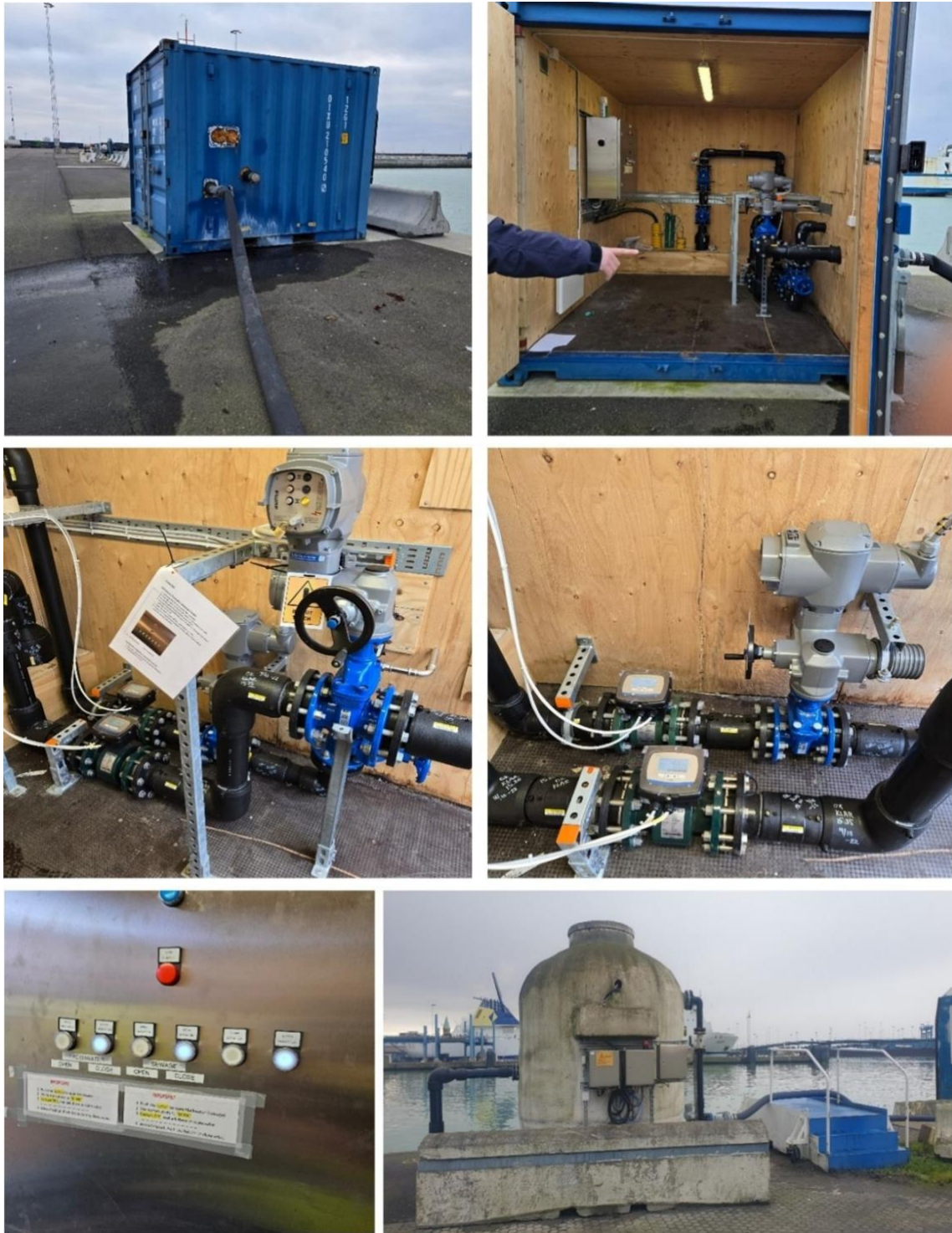
Figure 2: Port reception facility for blackwater and greywater at the Trelleborg Port.
