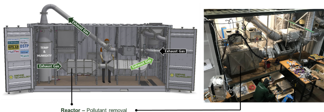
Figure 7. Scaled-up design (left) and construction (right) of Daphne's custom through-process exhaust gas monitoring system with Reactor to break down pollutant gases.
